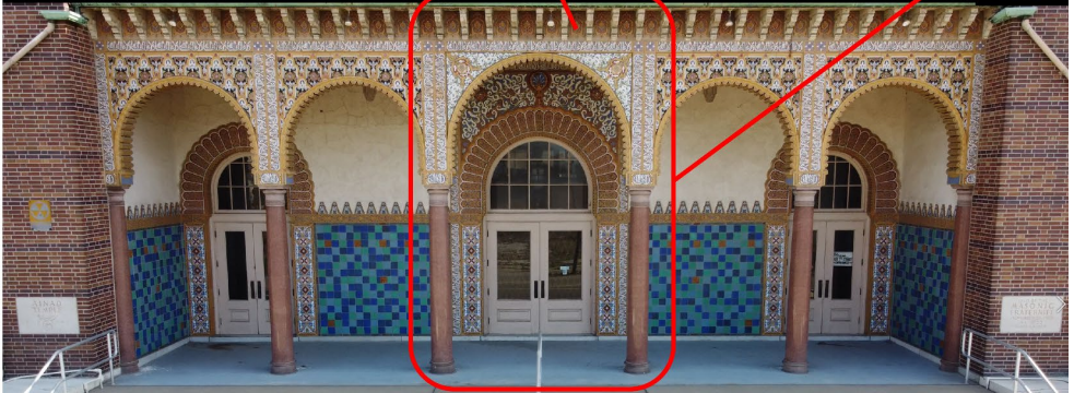
The middle image is the south elevation along St. Louis Avenue. The top row left image is the copper copula which is located in the tile roof above the loggia and to the right is the decorative terra cotta Shiner emblem which sits atop the parapet at the south façade above the main entrance. The bottom image is the loggia with polished granite columns, terra cotta detailing in addition to a ceramic tile wainscot. Note the signage to the left which indicated the fall-out shelter designation.
