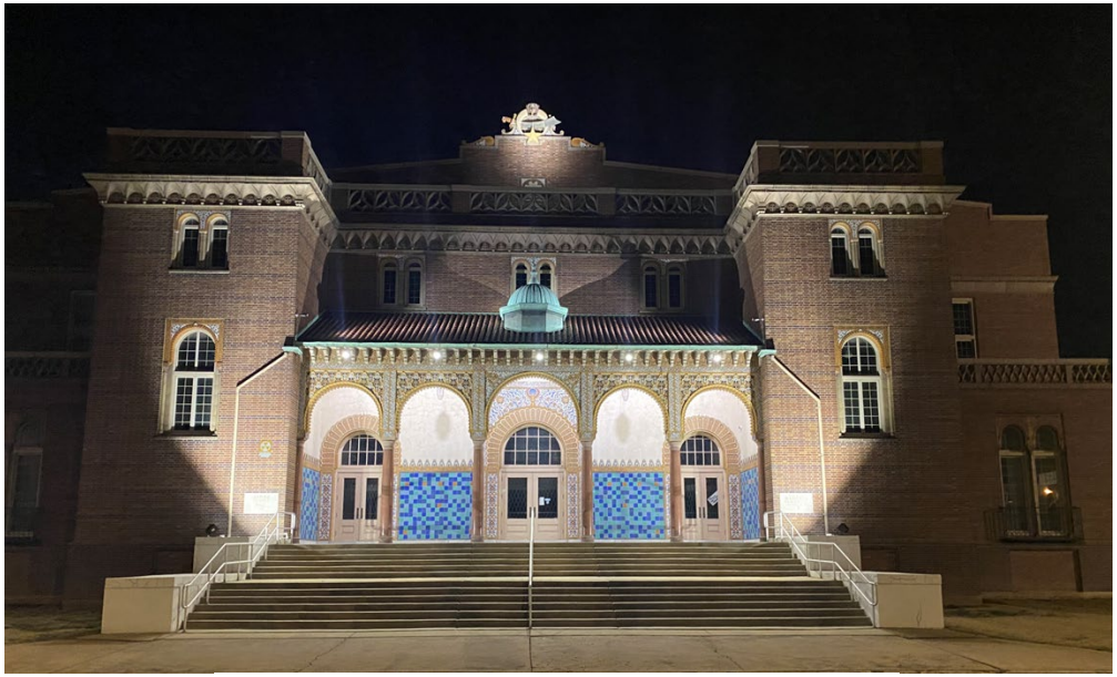
Front Elevation / South Façade along St. Louis Avenue
